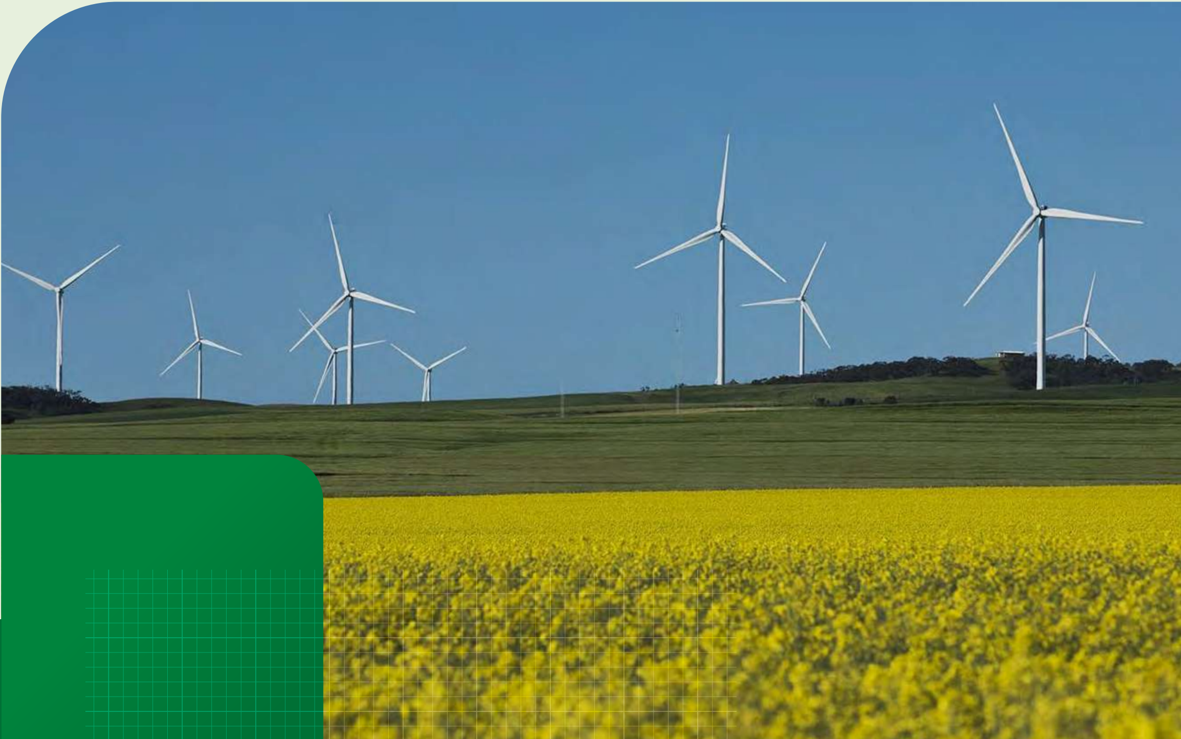
Hornsedale Wind Farm, South Australia
