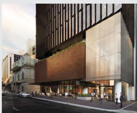
83 Pirie Street, Adelaide, SA Delivered as one of Australia's first all-electric office towers
